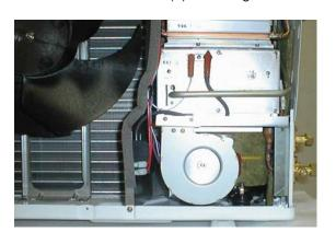
② Remove the screw (1) of the side cover, the screws (3) of the terminal block cover, and the screws (2) of the terminal block.
